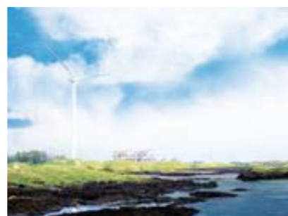
KIER wind farm in Jeju island.
